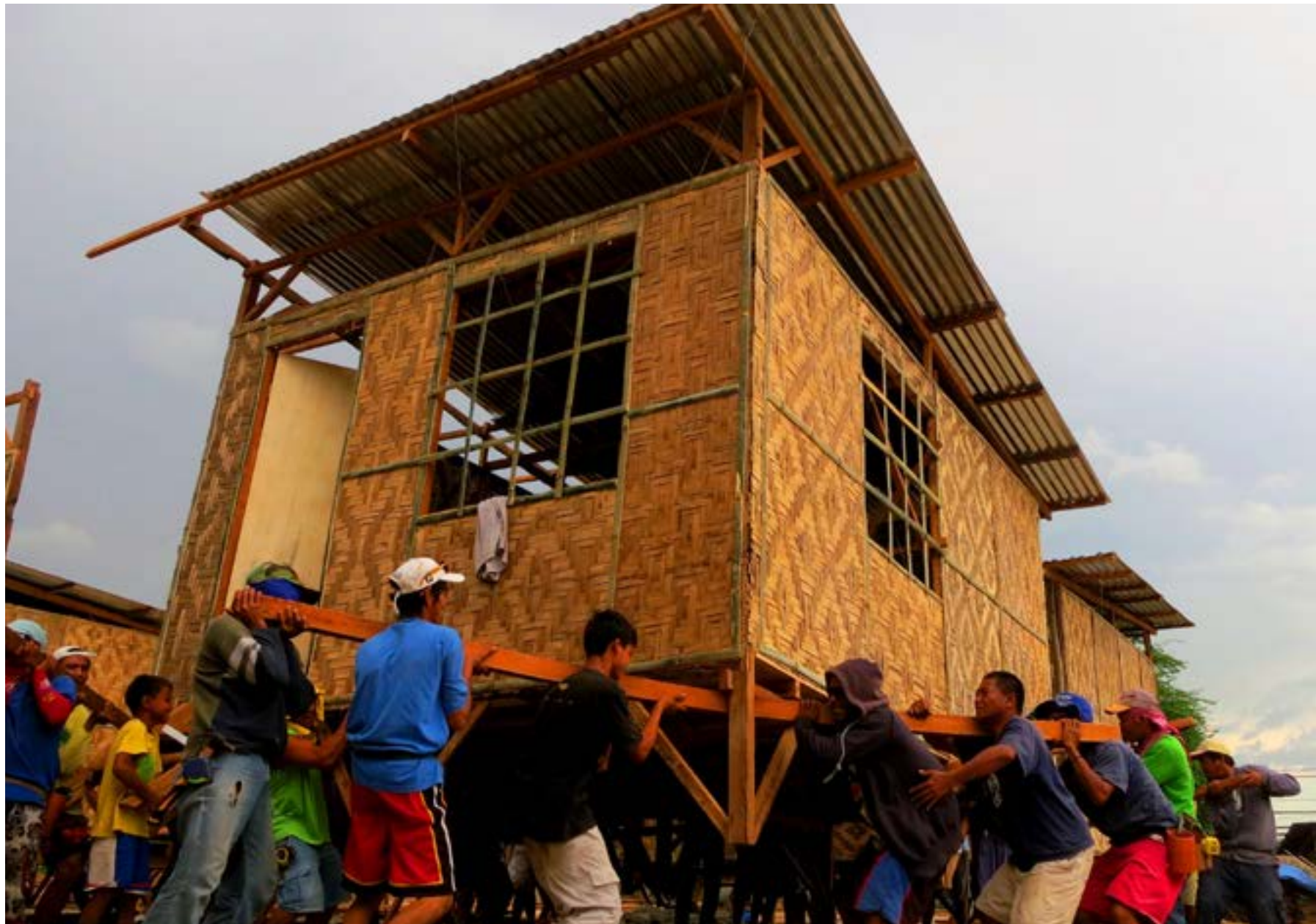
Moveable! Transitional shelters being moved by 20 people Photo by Charisse Mae Borja
