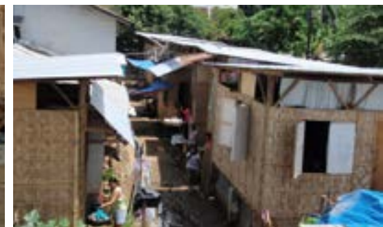
Urban transitional settlements by CRS in Cagayan de Oro City Photo by Seki Hirano/CRS
